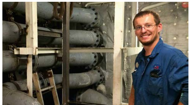
Onboard the PRIDE OF AMERICA - the Norwegian Cruise Lines ship which sails among Hawaiian islands. 1 st A/E Bryon Long shows off the new Exhaust Scrubber System piping which allows NCL to burn less expensive fuel while maintaining high environmental emission standards.
