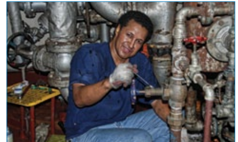
M.E.B.A. Engineer Luke Kaili gets ready for some engine room repairs during a Hawaii port stop aboard the SS MATSONIA.
