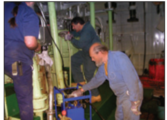
M.E.B.A. engineers Chris Butler and George Henderson pull a piston aboard the APL AGATE during its stop in Norfolk, VA in April.
